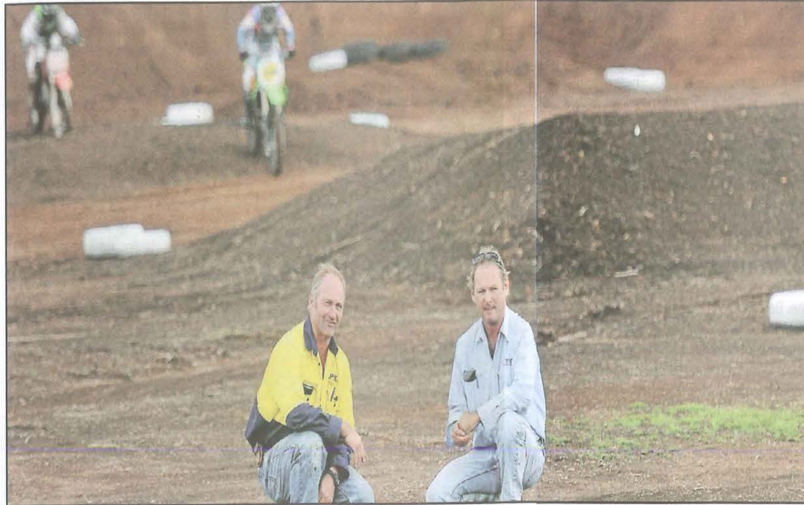
TPE foreman Mark Soper, left, a keen motorcyclist, put in plenty of his own time on the project, with TPE owner Bruce Chapman.
